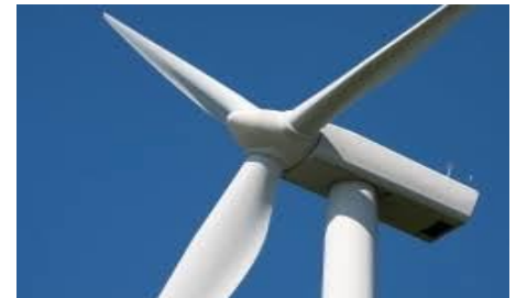
Fig 2C: Modern windmill with fiber reinforced blades
